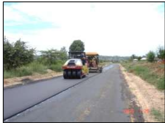
Photograph 6 Surfacing of the recycled base after being opened to traffic for two months
