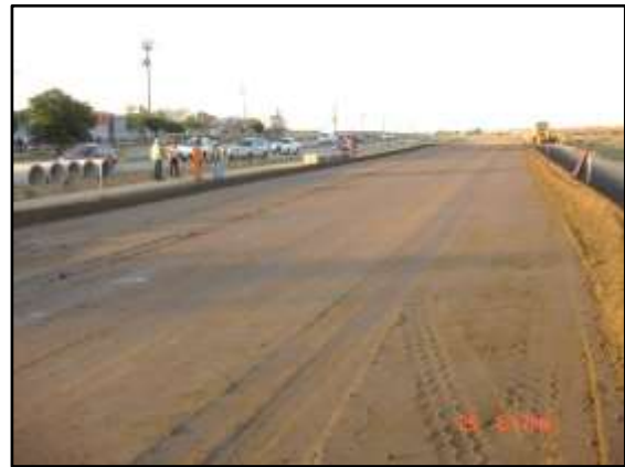
Photograph 3 Condition of trail section just before final roller passes
