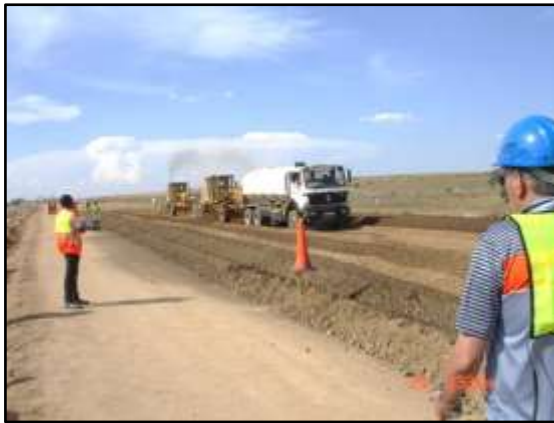
Photograph 2 Mixing of stabilising agent using a water cart and two graders
